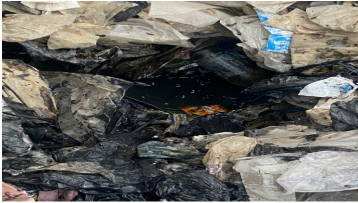
Figure 4: Leachate collection section of the Dumpsite at Mile 12, Kosofe LGA, Lagos State
